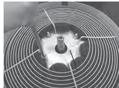
(9) Remove motor mounting nuts.
